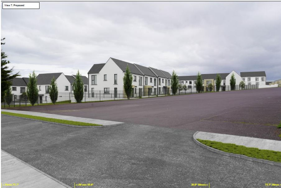
Figure 4. View from Delaneys GAA Car park
